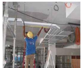
Cable trays and electrical trunking being installed. Across all levels, surface treatments and some finishes were applied.
