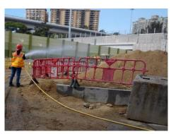
(ii) Cover stockpiles of dusty materials for backfilling with impervious sheeting when not in use.
