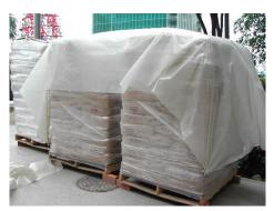
(ii) Carry out the de-bagging, batching and mixing processes in an area sheltered on the top and the 3 sides.
