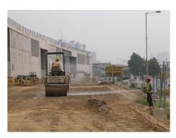
(iv) Treat exposed earth properly by compaction, turfing, hydroseeding, vegetation planting or suitable surface stabilizer.
