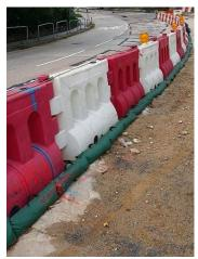
(xii) Seal the footing of hoarding to avoid seepage of surface run-off out of construction site.
