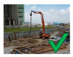
• Use non-percussive equipment such as hydraulic crusher, sawing, coring machines etc. for demolition and concrete breaking work.
