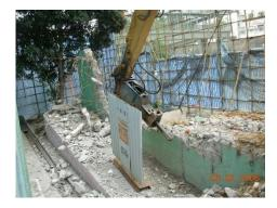
(ix) Totally enclose operation which emits dust and fine particles.
