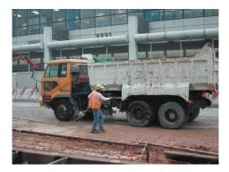
(vi) Cover the load of the vehicle which is carrying a load of dusty materials and leaving a construction site entirely by clean impervious sheeting to ensure that the dusty materials do not leak from the vehicle.
