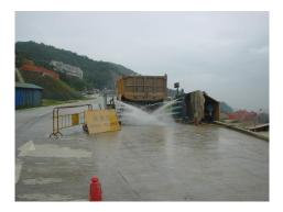
(iv) Regularly remove sludge accumulate inside the wheel washing facilities.
