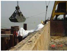
(v) Handle the dredged material with care to avoid splashing into surrounding waters during loading. Ensure the filling material is released below the water level.
