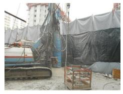
(iii) Use non-percussive pile driving methods such as vibration or jacking method for installing or extracting sheet piles.
