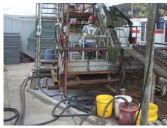
(iv) Provide perimeter channel to direct wastewater from grouting site to wastewater treatment facilities before discharging.
