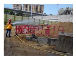
(ii) Spray water over the excavated material immediately before and during loading onto the dump truck.
