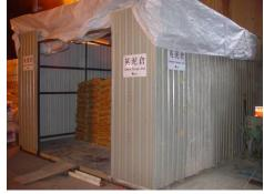
(ii) Carry out the de-bagging, batching and mixing processes in an area sheltered on the top and the 3 sides.
