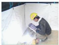
(viii) Provide screen to reduce dispersion of fugitive dust and particles.
