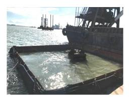
(vi) Use silt curtain to screen the marine work to control sediment suspension. The silt curtain should be fabricated from permeable, durable, abrasion resistant membrane like geotextiles and be mounted on a floating boom structure surrounding the grab and should extend to the sea bottom.
