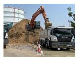
(iii) Do not load the materials to a level higher than the side and tail boards of the vehicles.
