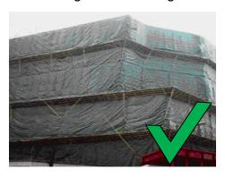
• Enclose debris chute and collection chamber by dust screen.
