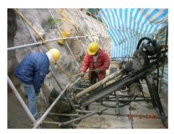
(v) Erect dust screen around the working area to reduce dust emission.
