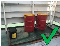
• Ensure that designated chemical storage and chemical waste container be enclosed on at least 3 sides by a wall, partition or fence with a height of not less than 2 metres or the total height of containers in stack, whichever is less.
