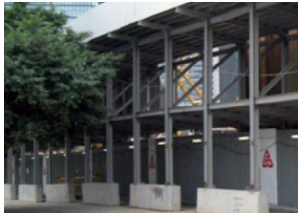
Erecting double deck hoarding for building construction work.
