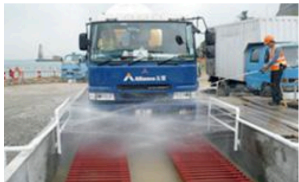
Using automatic wheel washing facility for vehicle cleaning.
