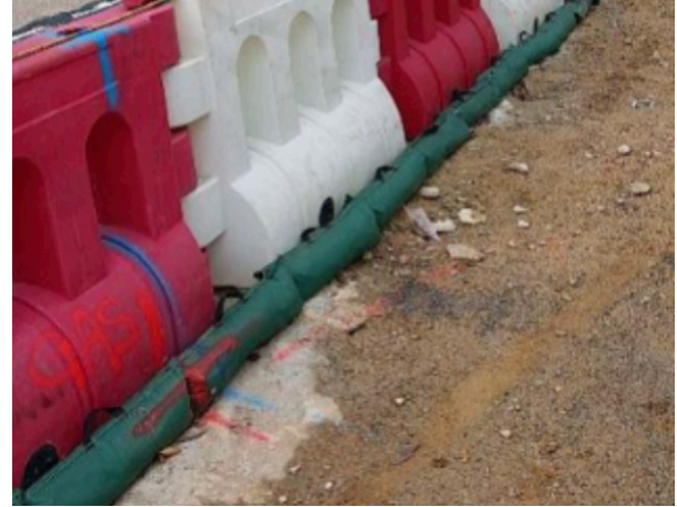
Providing earth bund/channels at site boundaries to intercept surface runoff from leaking out of the site.
