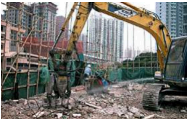
Using hydraulic concrete crusher for demolition works.
