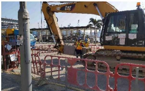
Adopting hammer bracket (the bracket made of special alloy lined sound insulating material) to reduce the noise from excavator-mounted breaker.
