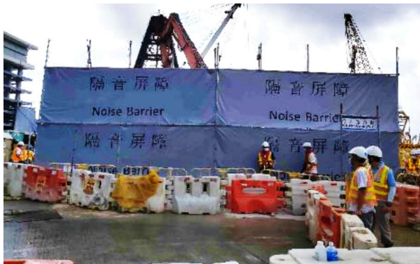
Erecting noise barriers to screen demolition activities.
