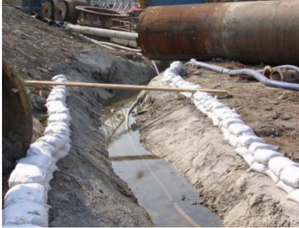
Providing earth bunds / channels to divert site runoff and wastewater to wastewater treatment facility.
