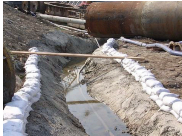
Providing earth bunds or geotextile for gullies to prevent discharging surface runoff without desilting.
