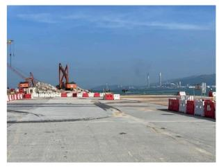
Main haul road shall be paved with concrete, bituminous materials, hardcore or metal plates, and kept clear of dusty materials.
