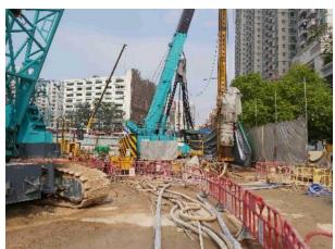
Spraying with water continuously and providing dust screen during drilling work.
