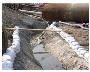
Providing earth bunds or geotextile for gullies to prevent discharging surface runoff without desilting.
