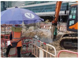
Dampening the breaking surface to suppress dust during breaking work.
