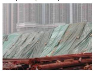
Covering dusty stockpile and exposed slope entirely by impervious sheeting to avoid windblown dust emission.
