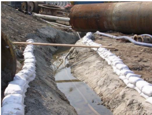
Providing earth bunds/channels to divert site runoff and wastewater to wastewater treatment facility.
