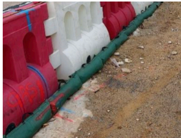
Providing earth bund/channels at site boundaries to intercept surface runoff from leaking out of the site.
