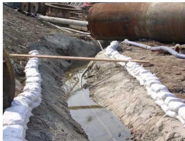
Providing earth bunds or geotextile for gullies to prevent discharging surface runoff without desilting.
