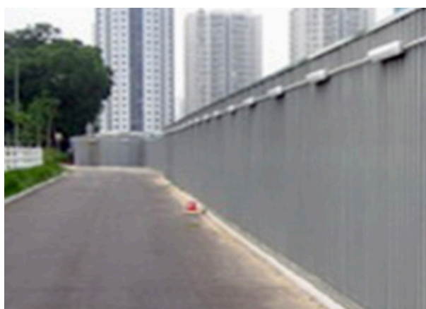
Erecting 2.4m high for site hoarding to act as a general barrier against construction dust dispersion.
